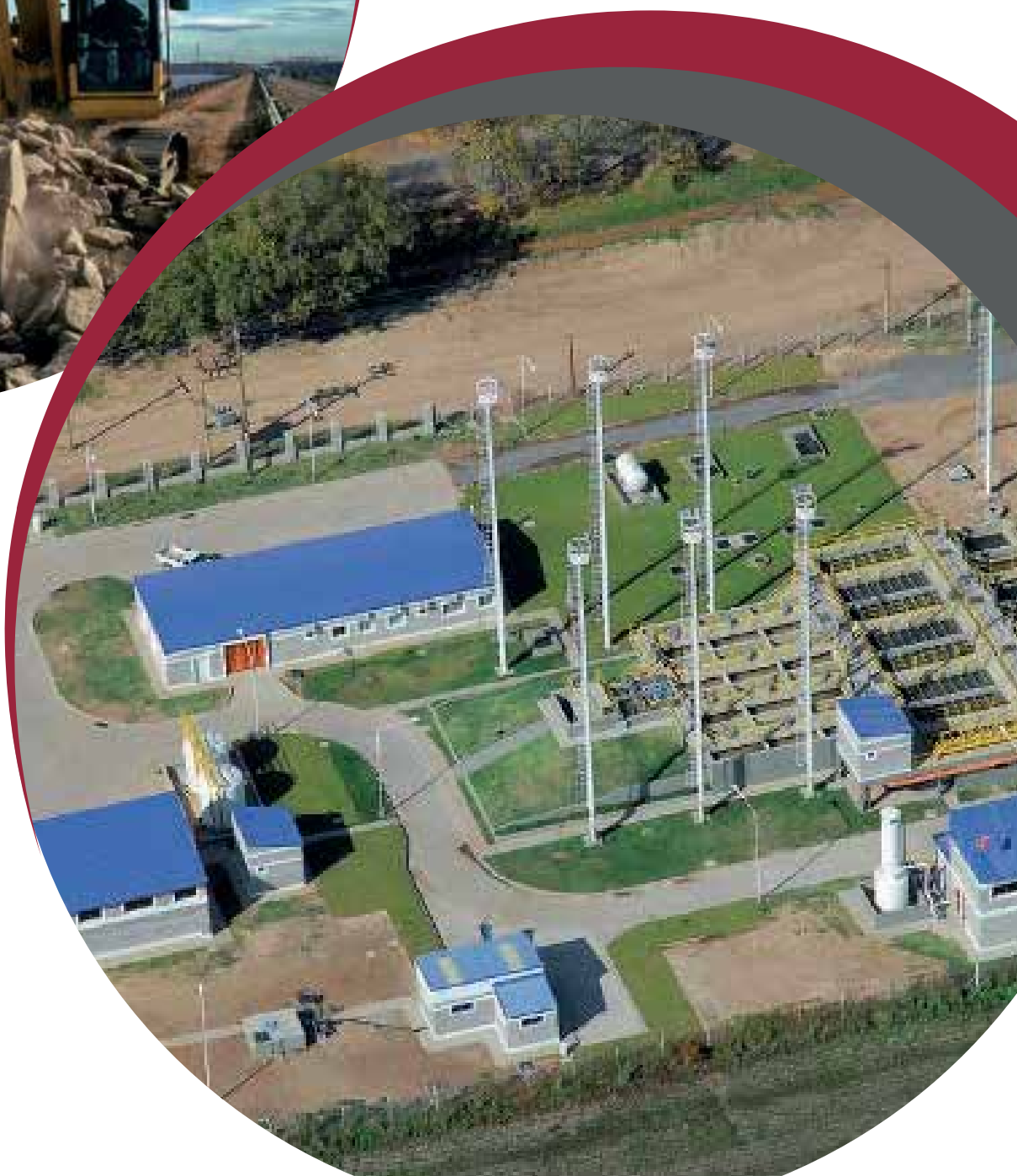
OBRAS DE INFRAESTRUCTURA / INFRASTRUCTURE WORKS
